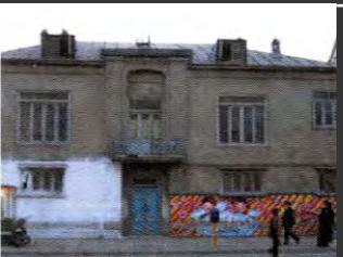
5 Building with open space access from closed space
