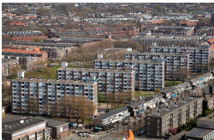
Figure A1.3:BoTU Gijsinglaan buildings (BAMwonen.nl)
