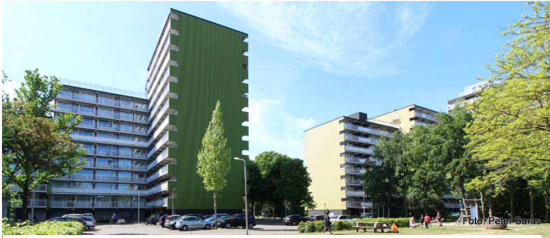
Figure A3.2 Renovation building Zwanenveld (Deduikenburger.nl)
