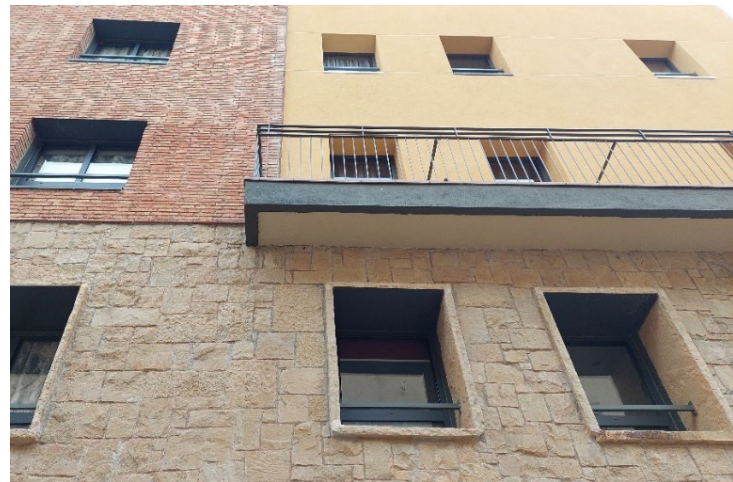
Figure A 7.2: Close up facade building (Redwell.com)
