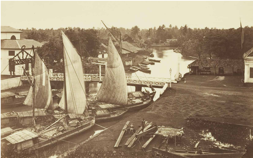
FIG. 3.10 Photo of seven pirogues in Batavia around 1872. This was the type of vessel that was used on a large scale for the river and coastal transport of coffee beans from Priangan to Batavia in the eighteenth and nineteenth centuries. Those in the photo belonged to the Bataviaasch Prauwenveer. This entity carried out the coffee transport along this route in the second half of the nineteenth century.
