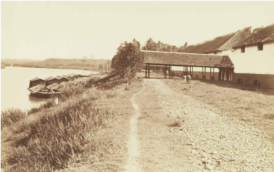
FIG. 3.8 The coffee warehouse next to the Ci Tarum near the settlement of Tjikao. The pirogues waiting for cargo belonged to the Bataviaasch Prauwenveer (BPV), the organisation that managed the shipment of the coffee to Batavia.
