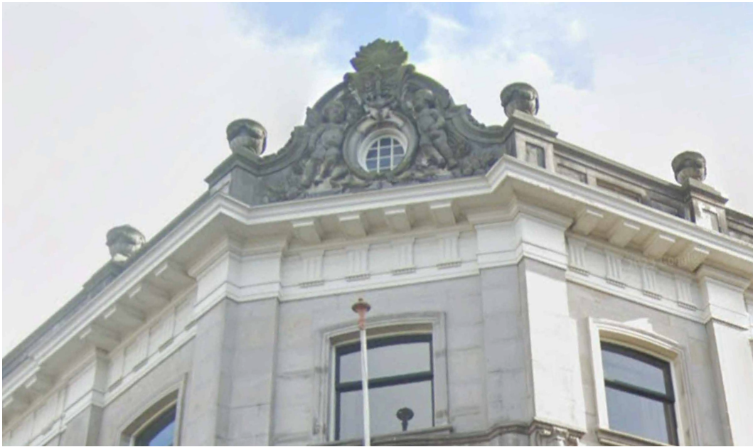
FIG. 4.39 Photograph of the roof façade of the head office of the Dutch Trading Society between 1858 and 1926. At the very top, one can recognise the anchor belonging to this organisation's trademark.
