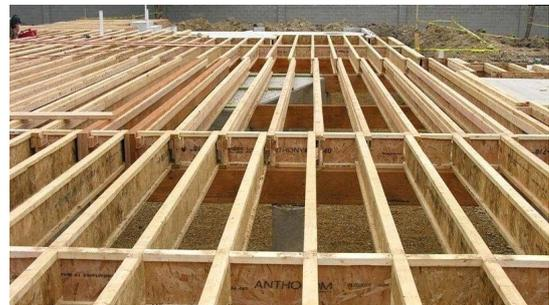
(b) I-joists as beams for flooring [33]
