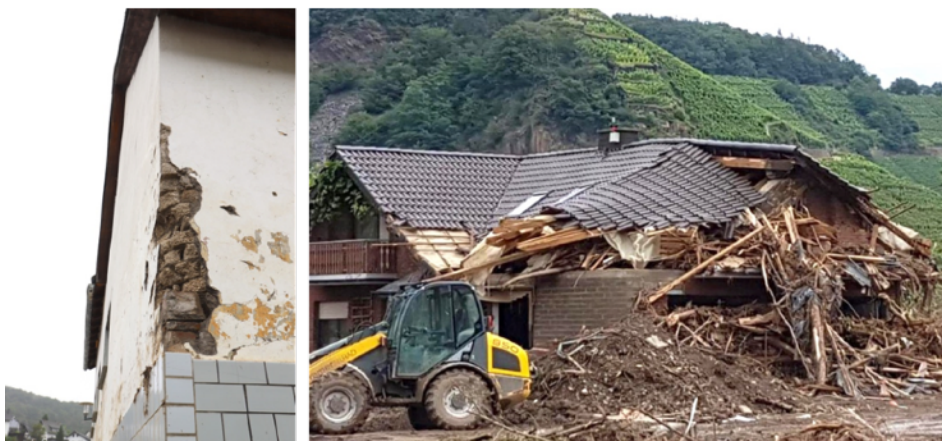
Figure A.8.1. Left, marks induced on buildings by debris impact, and right, debris damming around building openings.
