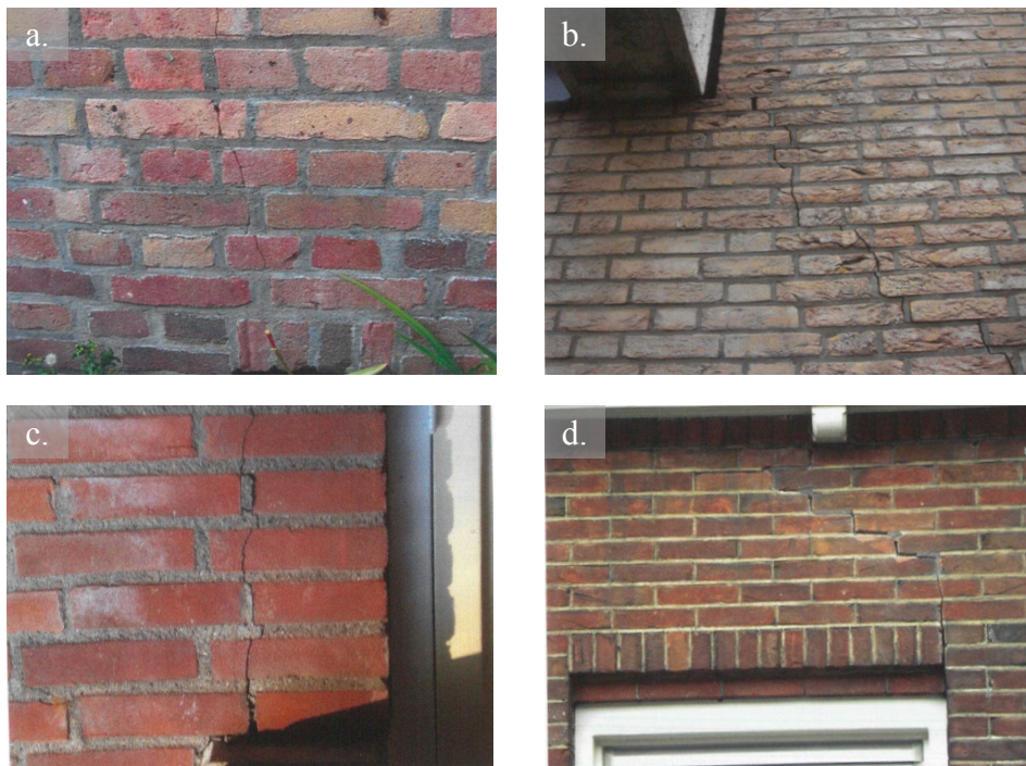
Figure 2.2.0. Photographs of cracks in bare masonry walls. (a) Small crack narrower than 0.5 mm; (b) crack approximately 2 mm wide; (c) crack narrower than 2 mm; and (d), wider than 5 mm. Adapted from [SBR].
