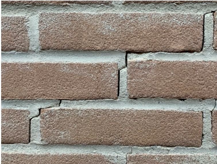
Figure 1.1.1. An example of a narrow crack in fired-clay brick masonry with a stretcher pattern and a cementitious general-purpose mortar in 10mm bed and head joints. This photograph was obtained from an experiment on a wall (see Chapter 3).
