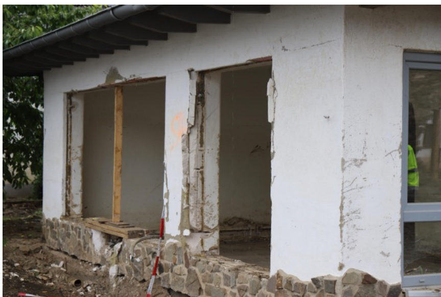
Figure A.8.2. Example of a façade where the flow of water and floating/trapped debris removed windows and knocked out a pier.
