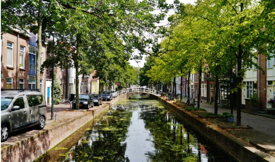
Figure 1. Old city-canal in Delft with masonry quay walls and a masonry overpassing with abutments.
