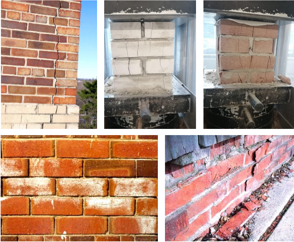
Figure 2.1.1. Examples of expressions of damage in masonry. a) A crack at the corner of a structure. b) Fine vertical cracks in the masonry due to excessive compression (crushing). c) Blistering on the bricks and the mortar due to efflorescence of salts. d) Serious scaling or delamination likely due to freeze-thaw cycles.
