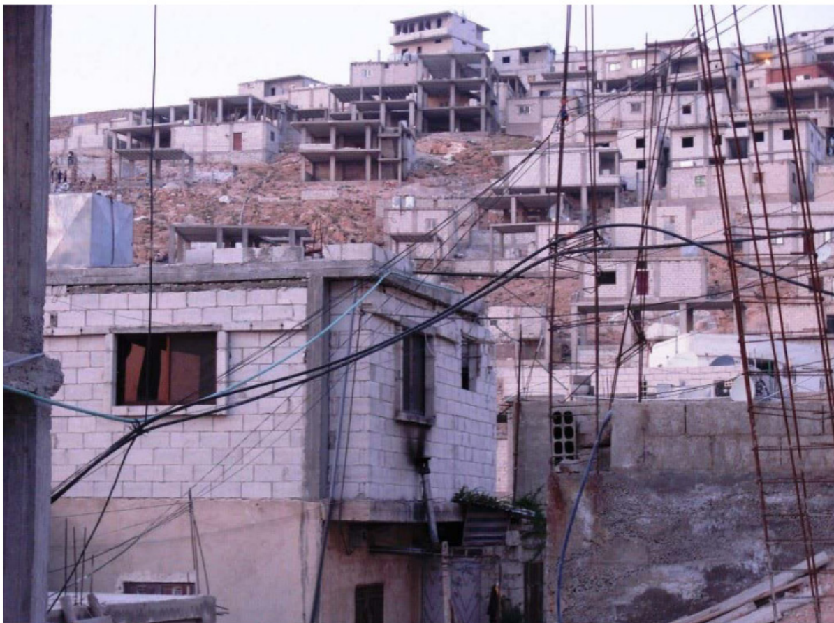
Figure 22 : Construction rebars of a house left exposed in an informal settlement (Kafa, 2013)
