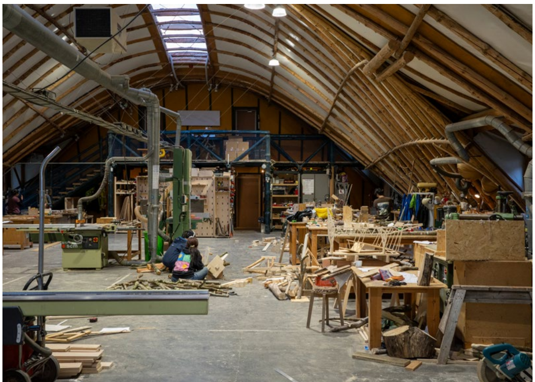
The roof structure of the main wood workshop, designed and built by Frei Otto. The buildings itself express the experimental programme of the site and dictate the use of wood. →
