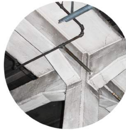
Grinnel system in the interior
