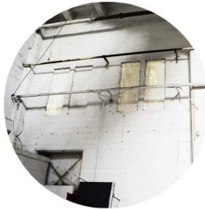
Grinnel system in the interior
