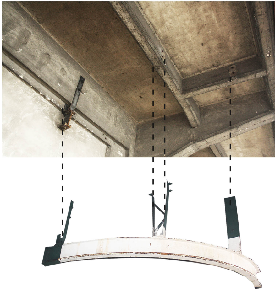
p.1 The tailor-made aspect of the Katoenveem's structure; the concrete beams were formed with wholes during the formwork in order to support the transit system
