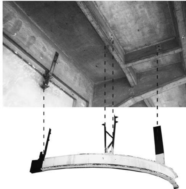
Pictures from the beams in the north part of the building; The wholes in the concrete beams are made during the formwork
