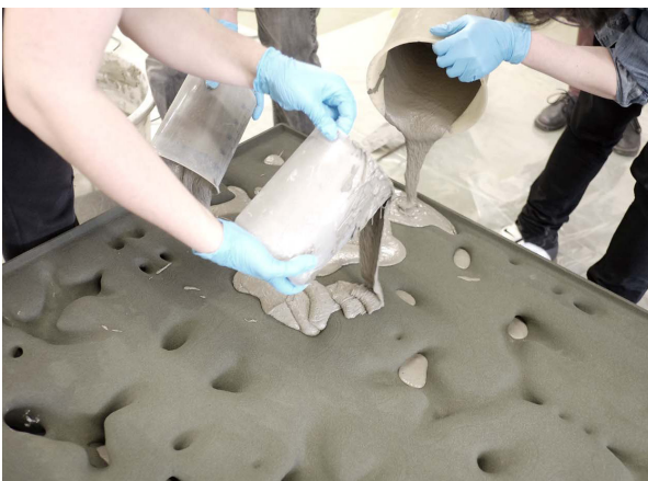
Image 13: Left: Element being constructed using the Stay-in-Place formwork technique. Right: Result 16
