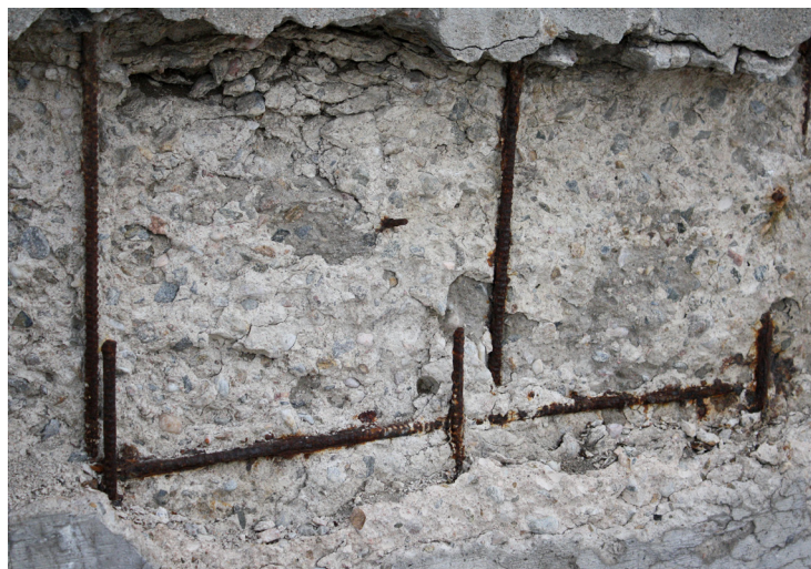
Image 6: Steel reinforcement inside a concrete element 9
