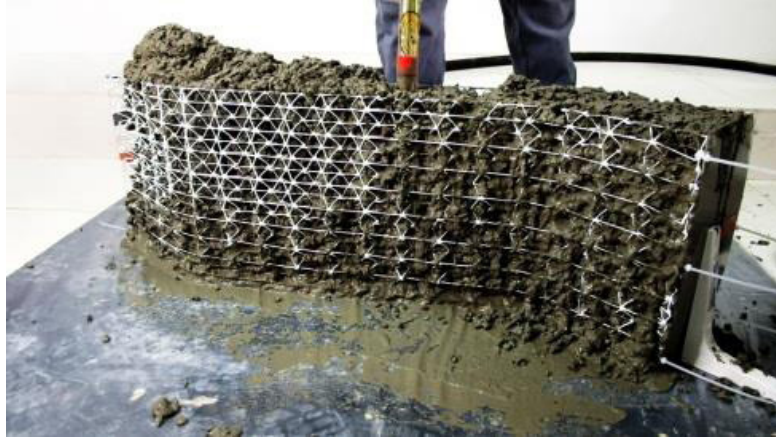
Image 12: Element being constructed using the Mesh mould technique 15
