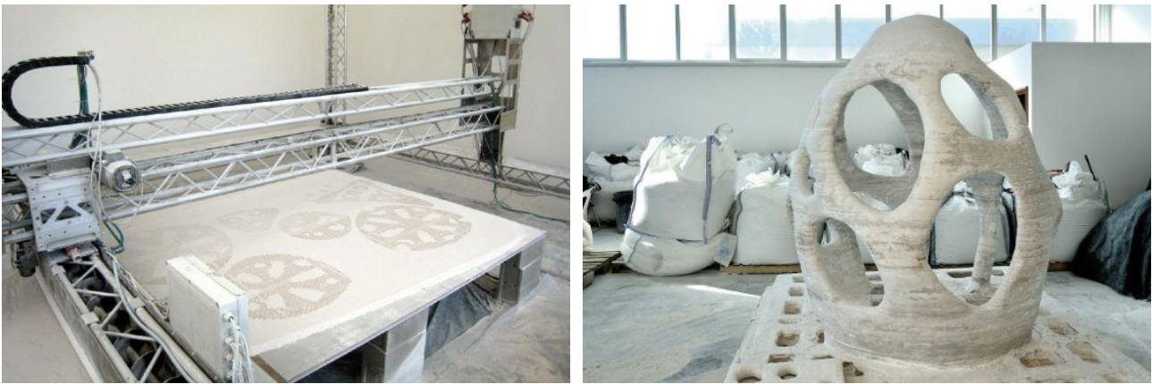
Image 8: Left: Element being 3D printed using the D-Shape technique. Right: Result 11
