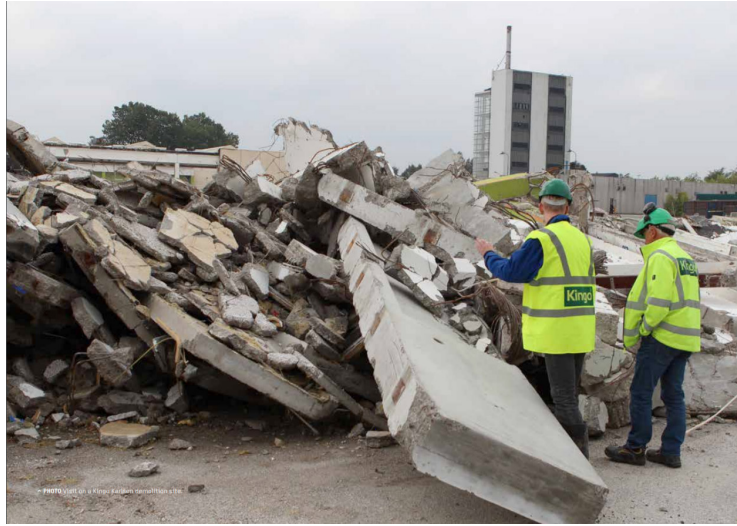
Image 1: Demolition site with piles of downcycled materials with low or no value as resources for future buildings 4
