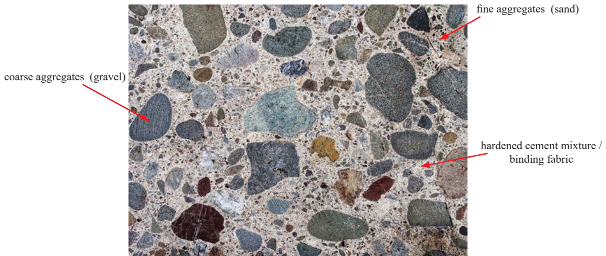
Image 2: Section of hardened concrete with its visible constituents 5
