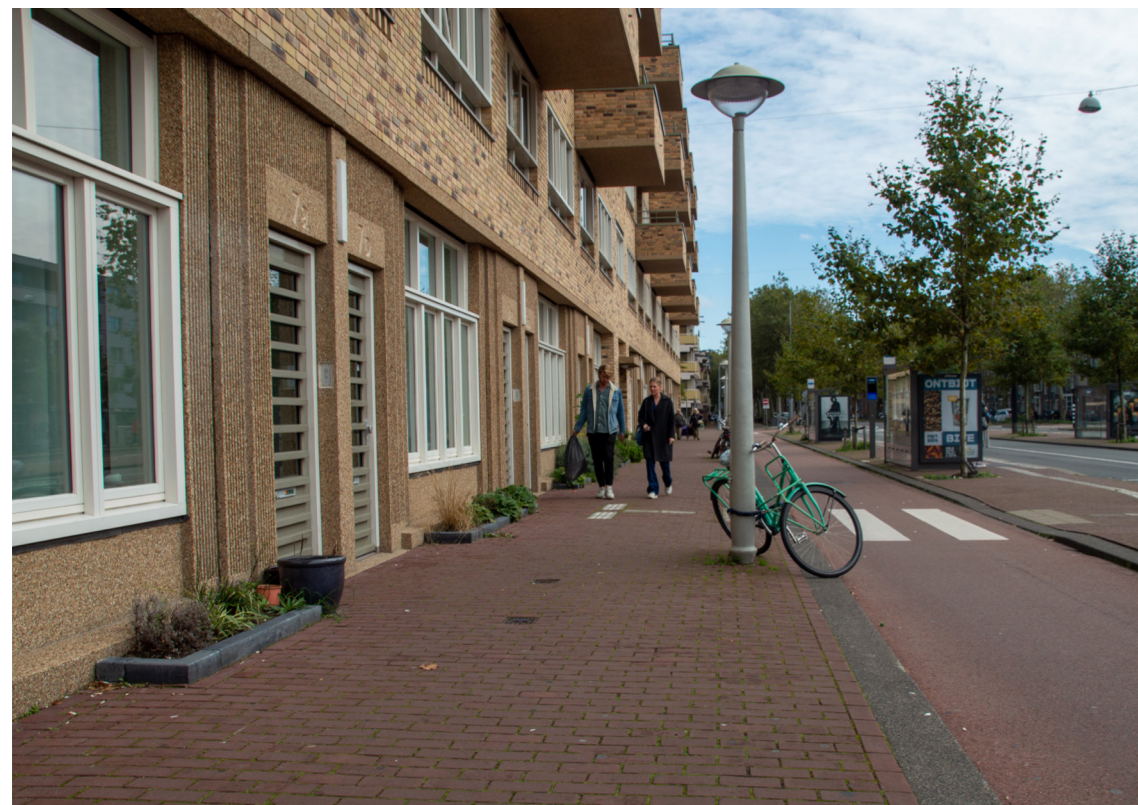
Figure 72: Renovated part of the Insulindeweg, Indische Buurt, Amsterdam (image by author, 2020)
