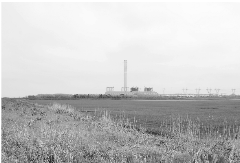
FIGURE 14.13 Porto Tolle power station. Source: Chiara Geroldi.
