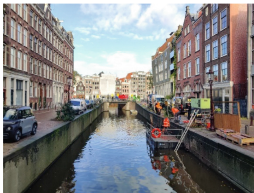
Fig. 1. A quay wall in Amsterdam
