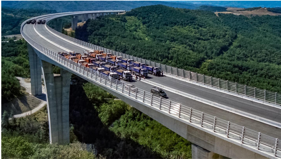
Figure 2. Example of diagnostic load test from Slovenia, 2008.
