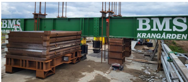
Figure 9. Partial testing of bridge slab, (June 2024, Denmark) (Schmidt et al., 2024).
