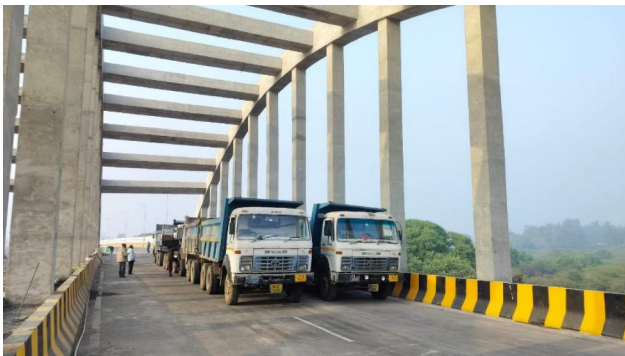
Figure 5. Example of load test in India.
