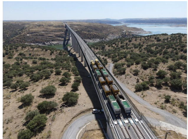
Figure 6. Load testing at El tajo Viaduct.
