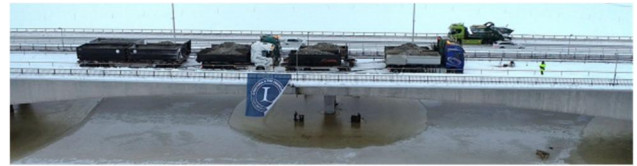
Figure 16. View of the midspan of the kalix bridge under proof loading.
