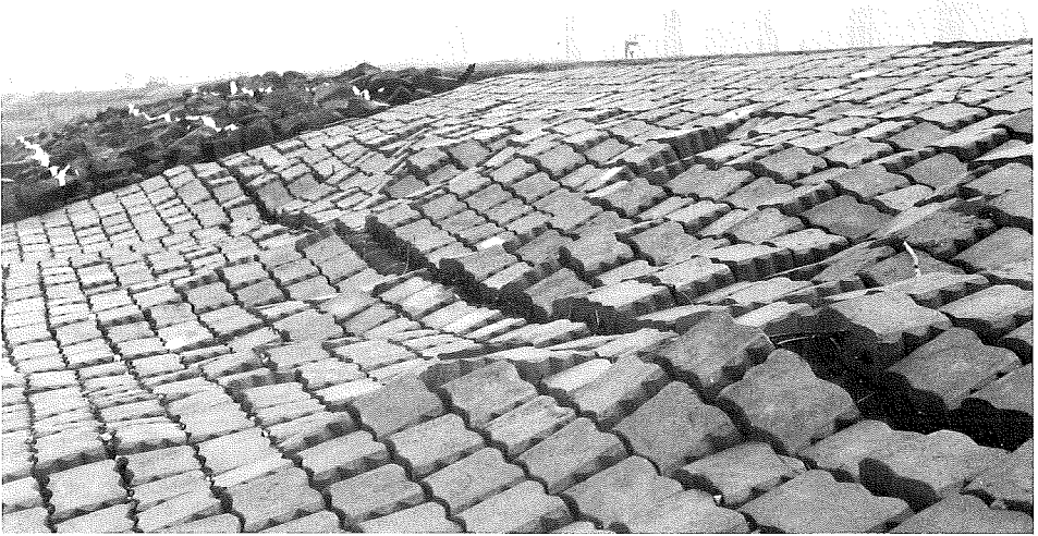
Fig. 18. Distortion of the surface of the slope caused by the movement of material under the mattress (test section near Lelystad).
