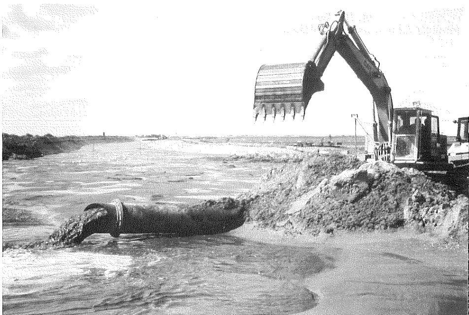
Fig. 80. Hydraulic filling with sand.
