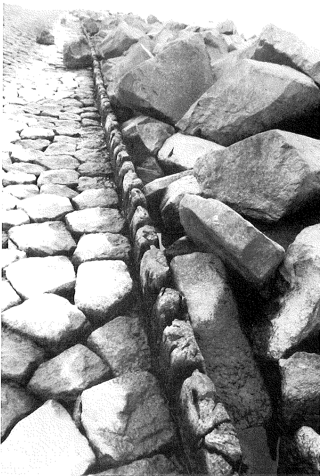
Fig. 145. Wooden toe structure (immediately before renovation).
