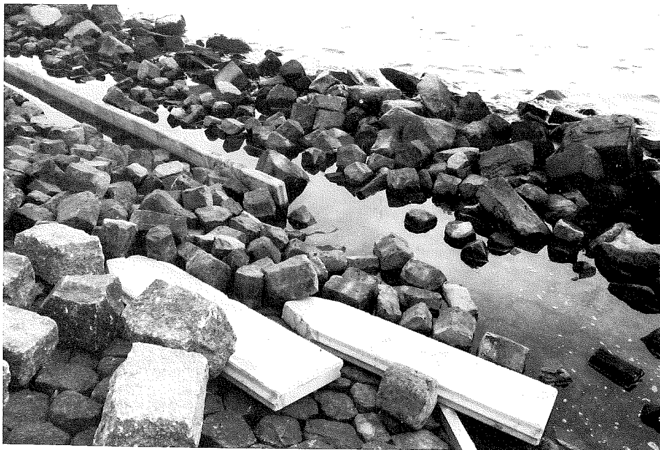
Fig. 144. Toe structure with concrete sheet piling (during renovation).
