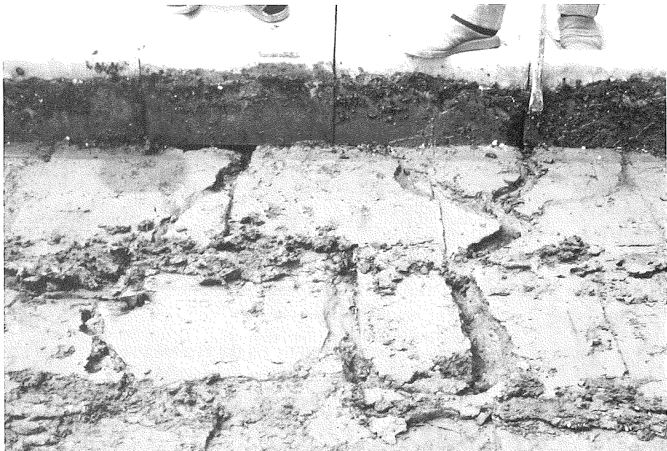
Fig. 30. Erosion channels in the surface of clay.
