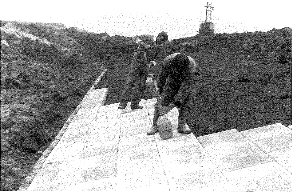
Fig. 84. Blocks being tamped-in.
