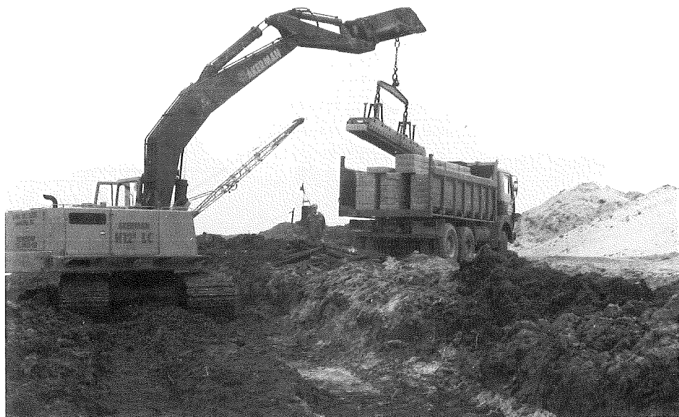
Fig. 82 Lifting a row of blocks with a block claw.
