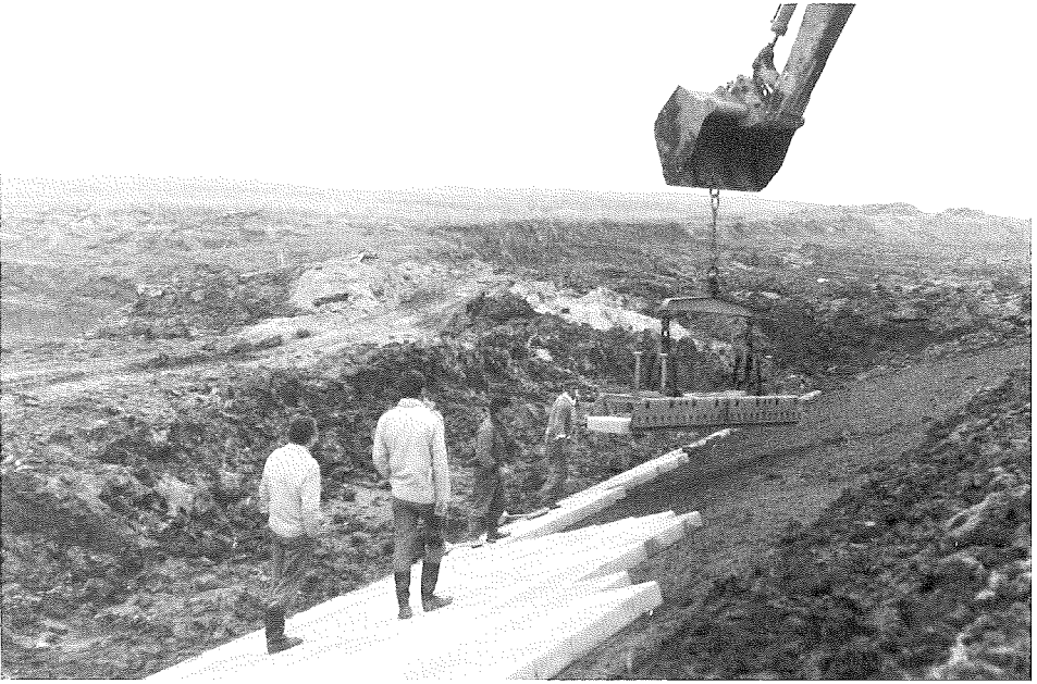
Fig. 83. Placing blocks with a block claw.
