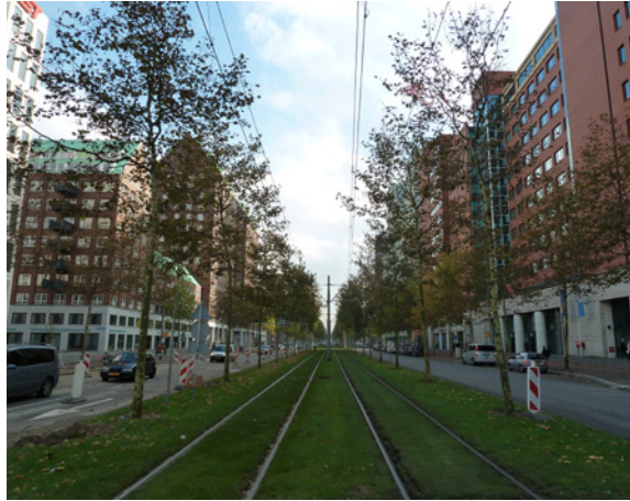
(top to bottom, left to right; all author's own) [6.20] railway tracks between Hillesluis (left) and Maaszicht (right) [6.21] buildings at Maaszicht block the view on the river [6.22] business real estate at Maaszicht [6.23] Laan op Zuid and the intersection with Varke-noordseviaduct [6.24] Laan op Zuid looking south [6.25] Hilledijk surrounding Afrikaanderwijk on the east and north sides [6.26] Hilledijk [6.27] Parkstad area seen from the south
