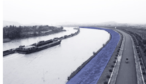
Ring dike along the Taihu lake
