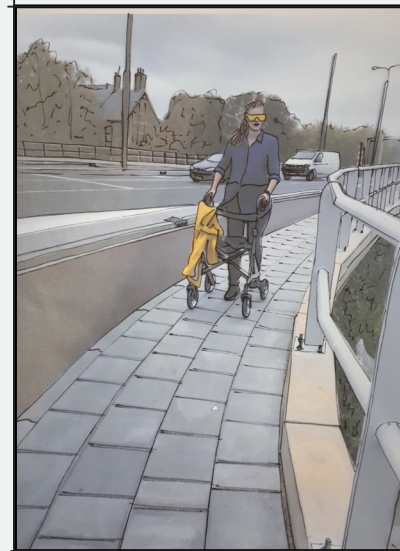
The slope of the bridge is too steep, the walker rolls away.
