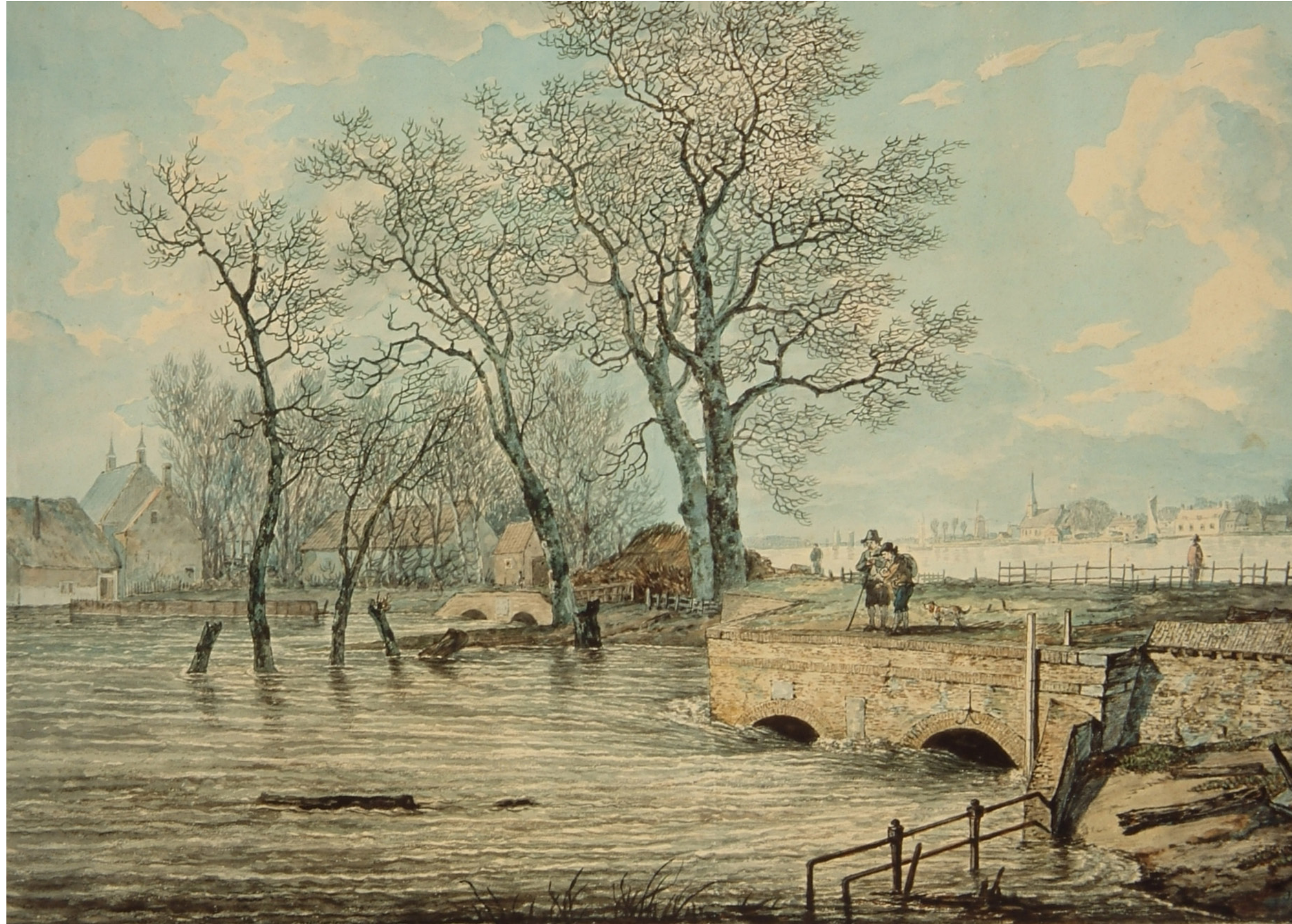
Near the sluices
