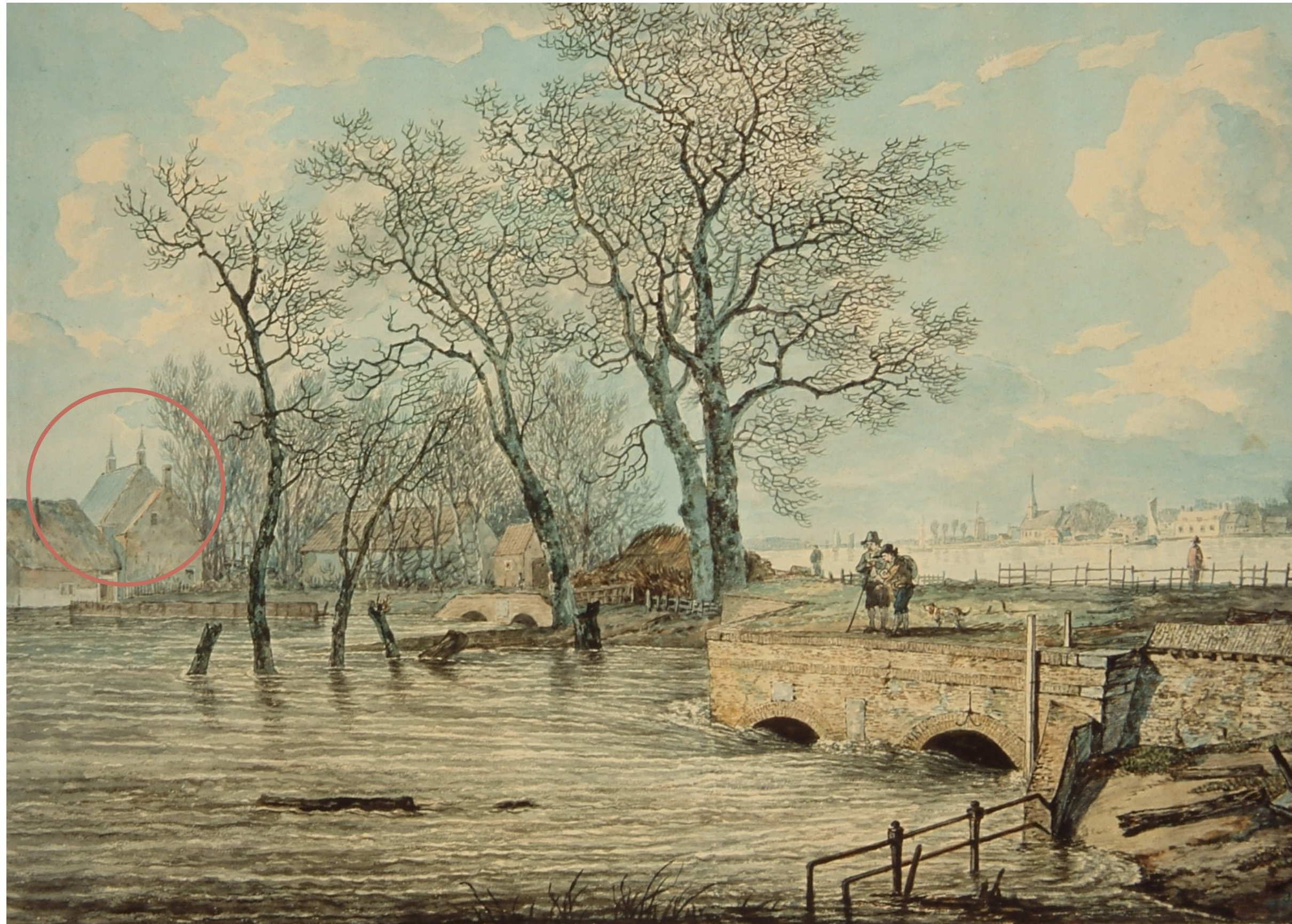
Near the sluices
