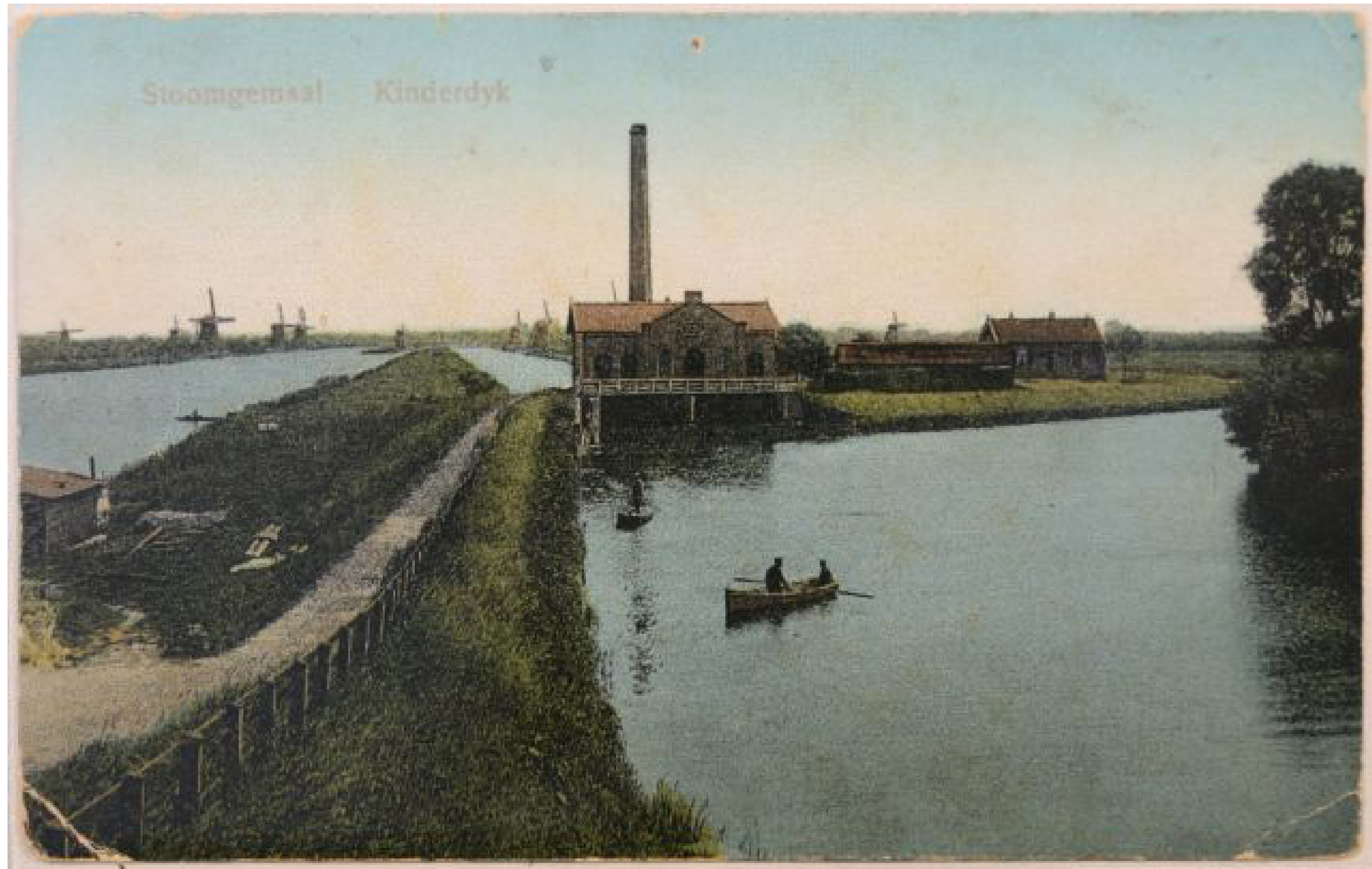
Steam pumping stations
