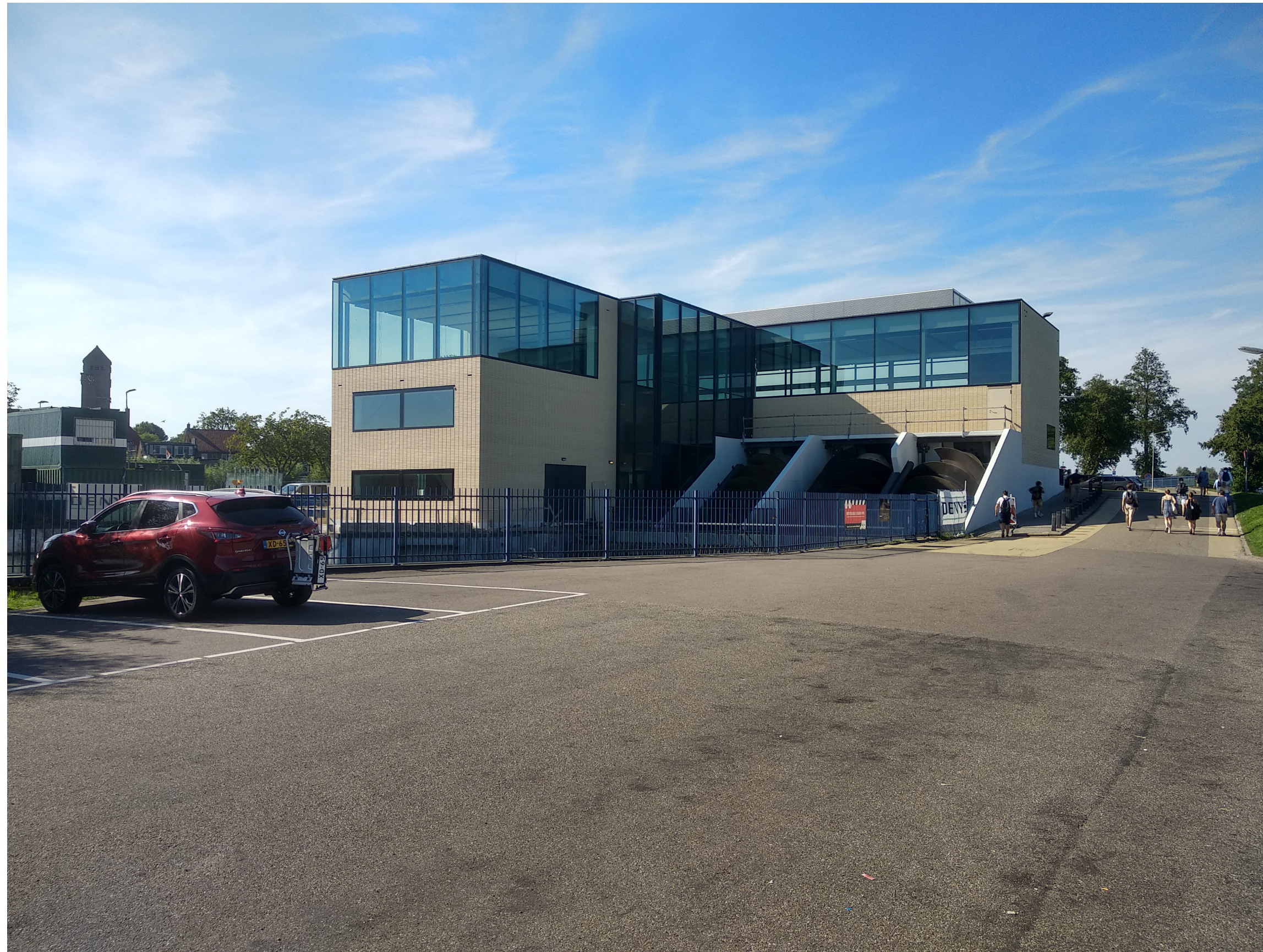
Diesel and electric pumping stations
