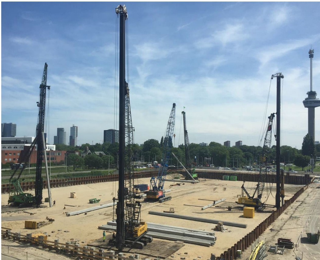
Figure 29: Five pile drivers are busy with the foundation of Little C (ERA-Contour, 2021)
