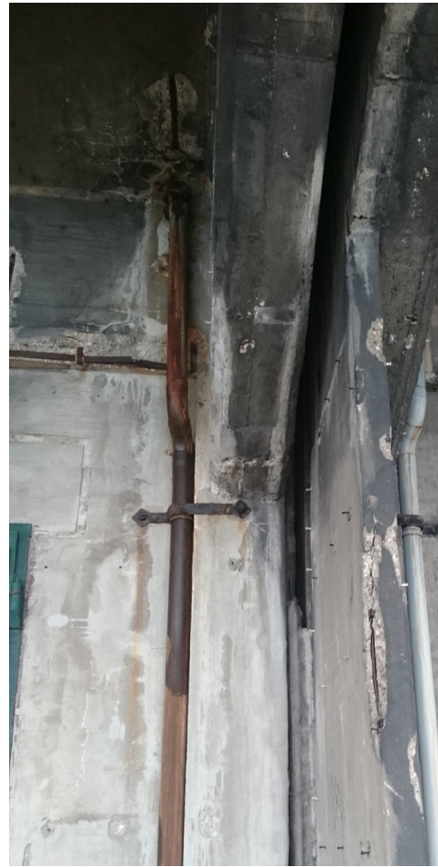
Fig. 78. Drainage pipes from roof on balconies
