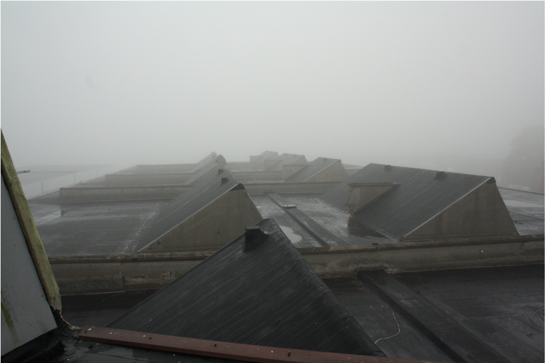
Fig. 96. The current situation on the roof, source: photograph by C. de Boon
