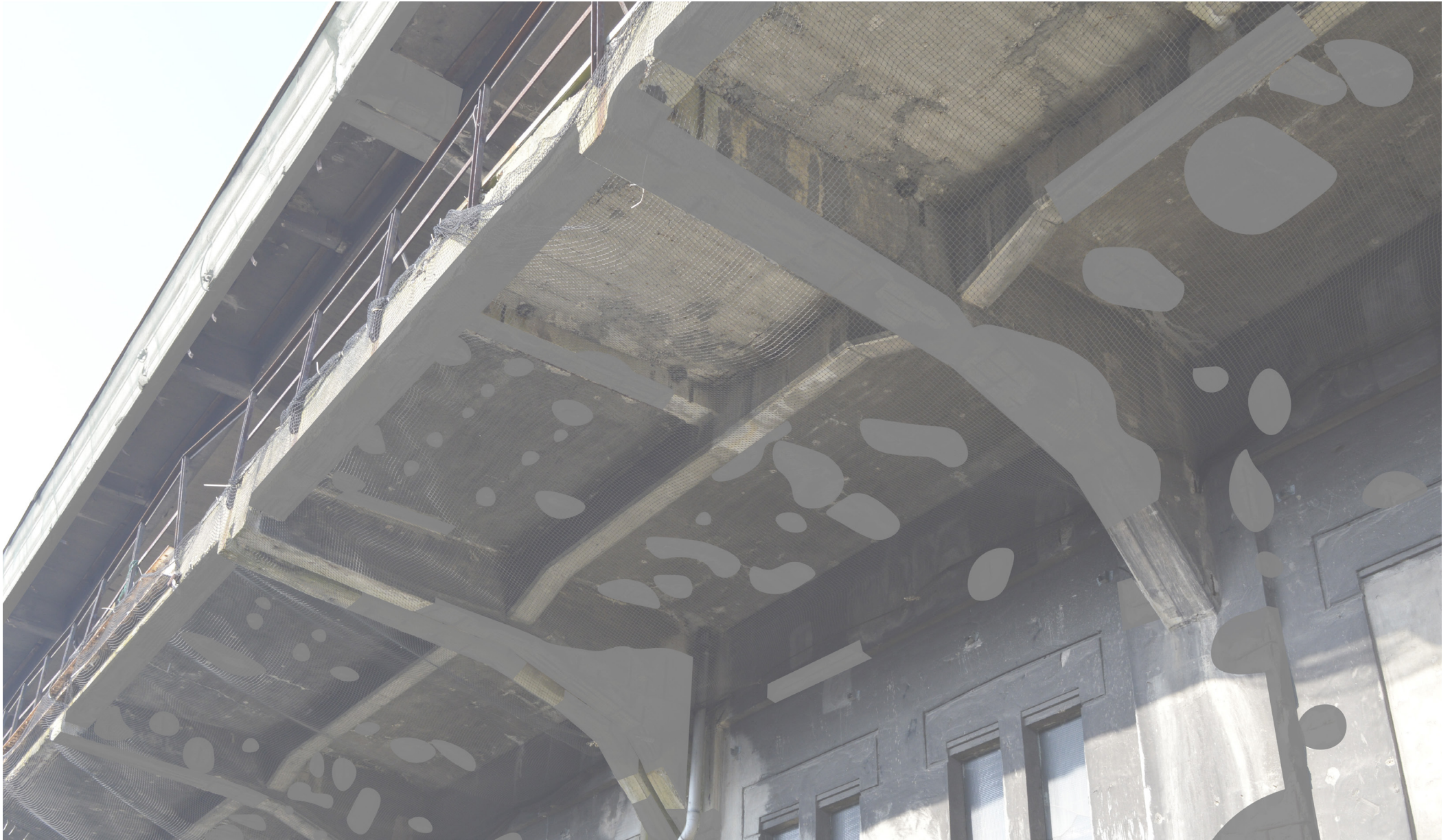
Fig.76. Repaired state of the facade, source: photograph by A. Loeff, edited by I.Louer
