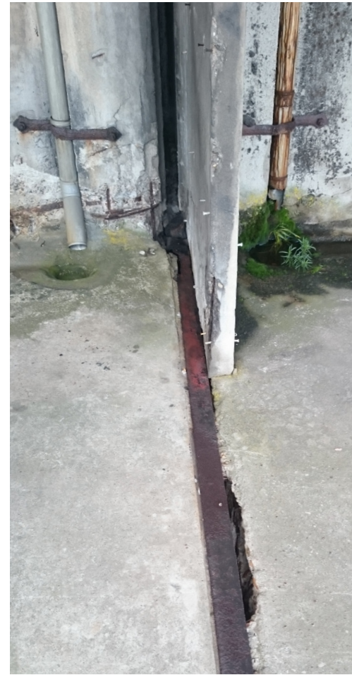
Fig. 79. Connection of drainage system through balcony floors
