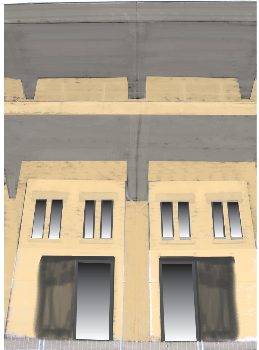
Fig. 161. Visualisation of Katoenveem with a reconstructed artificial sandstone render layer on the facade, source: photograph by C. de Boon, edited by I. Louer
