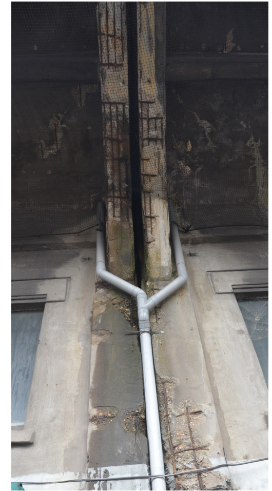
Fig. 80. Drainage pipes from the balconies
