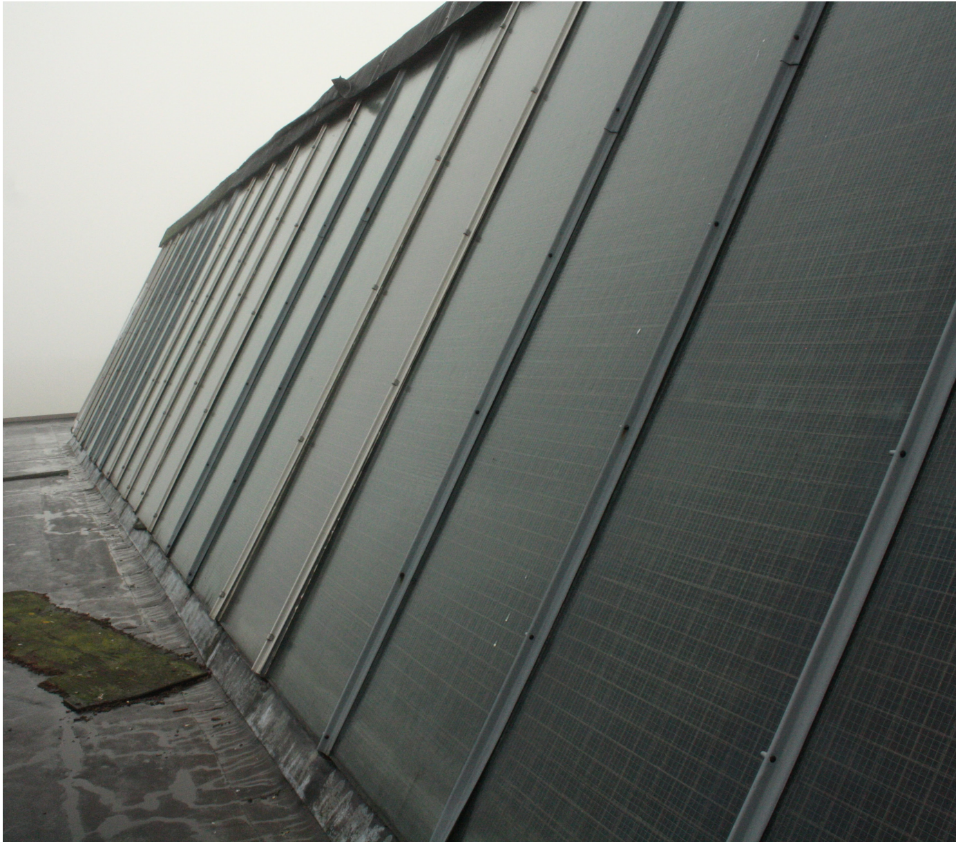
Fig. 83. Current state of the rooflights, source: photograph by C. de Boon
