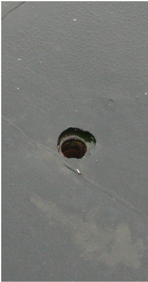
Fig. 77. Drainage opening on the roof
