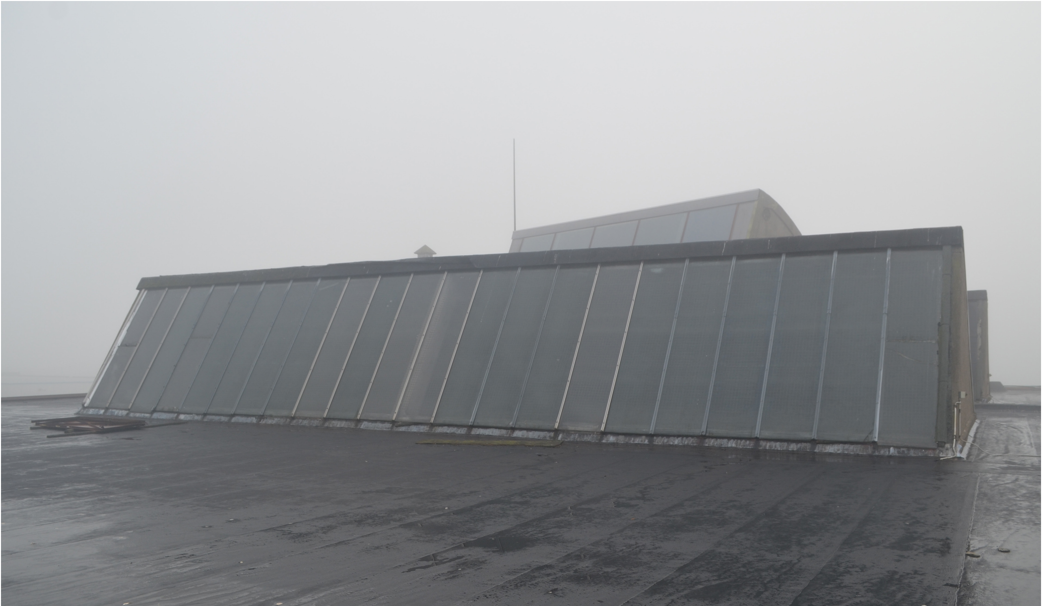
Fig. 87. Current situation on the roof, source: photograph by C. de Boon
