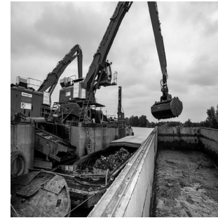
Dredging soil (afdekshop 2024)
