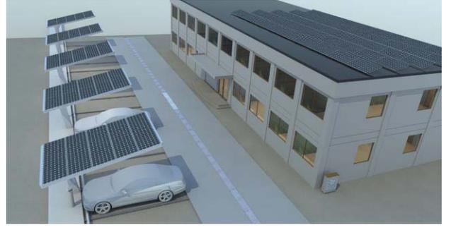
Fig. 1. EV charging powered by solar panels on roof and carport.
