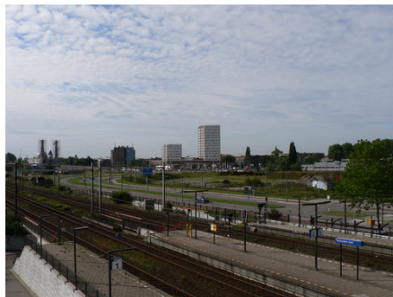
Train station Rotterdam Zuid Source: Panoramio.com
