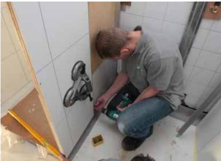
Renovatie badkamer/toilet (Bron: Faay)
