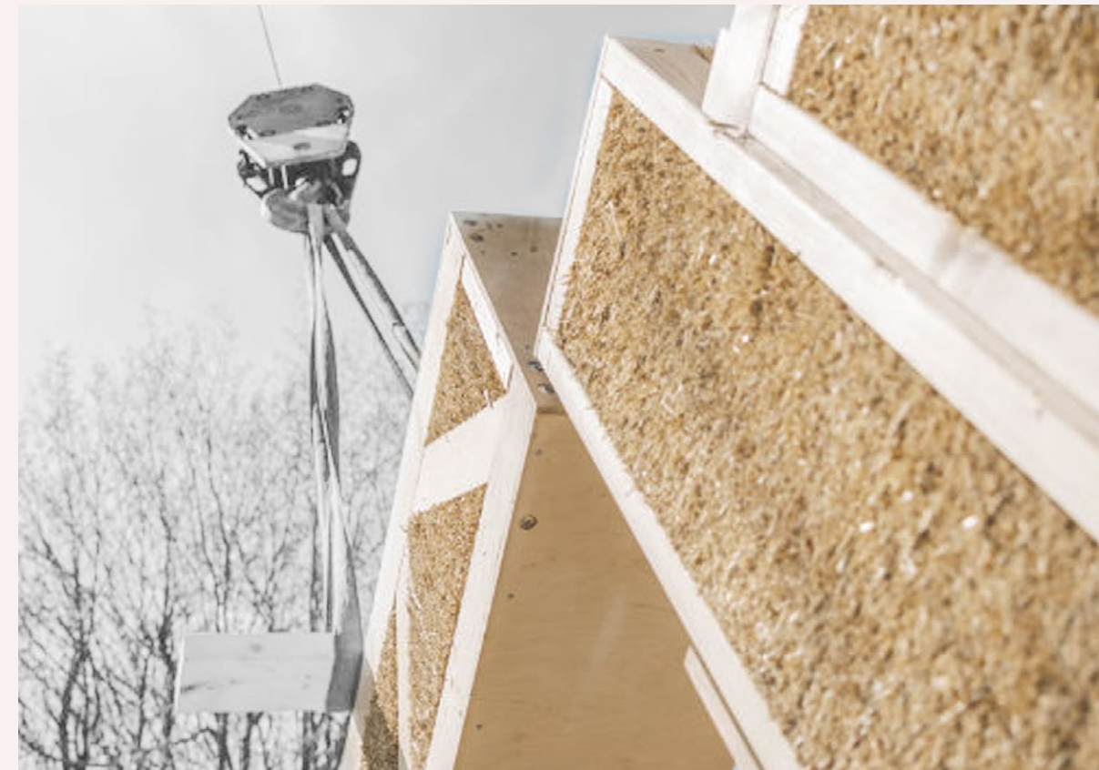
Figure 52: Prefab straw wall panels Source: EcoCocon
