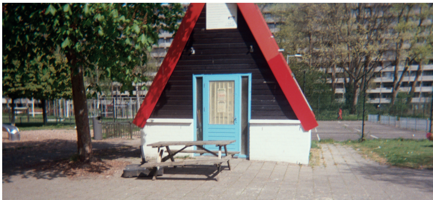
Figure 43. House on the playground (own work)
