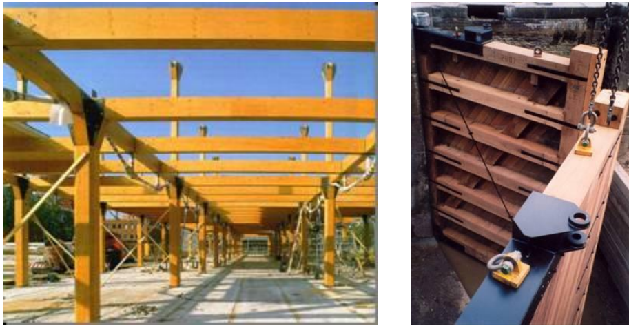
Figure 1.3. An industrial building from glued laminated softwood timber (left) and lock gate doors from tropical hardwood timber (right)
