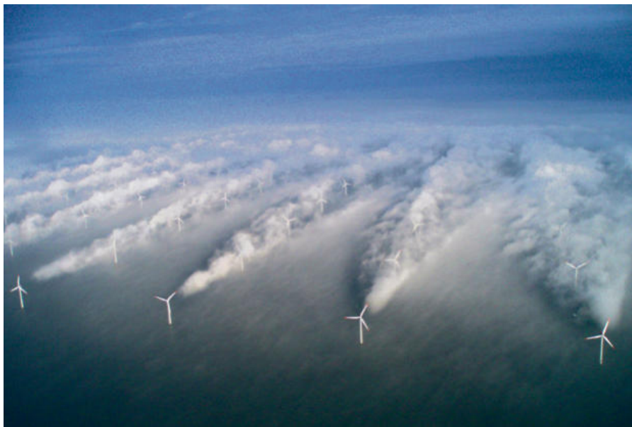
Figure 3.2: Turbine wake clouds at Horns Rev Wind Farm. Source: Emeis (2010), owned by Vattenfall, photographer Christian Steiness
