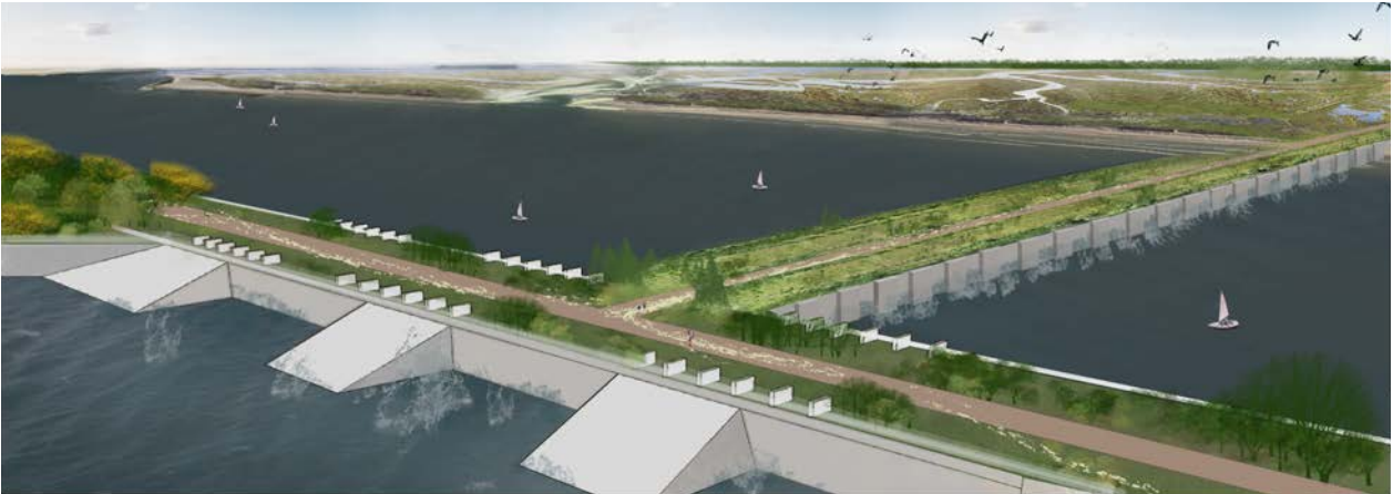
FIG. 1.81 Transition zone creek - eco-spillway and eco- bridge At this point many flows merge. The spillway and bridge are both infrastructure for people and animals. The bridge connects Voorne to Goeree and is therefore an alternative route for the Haringvlietdam and provides a new ecological corridor.
