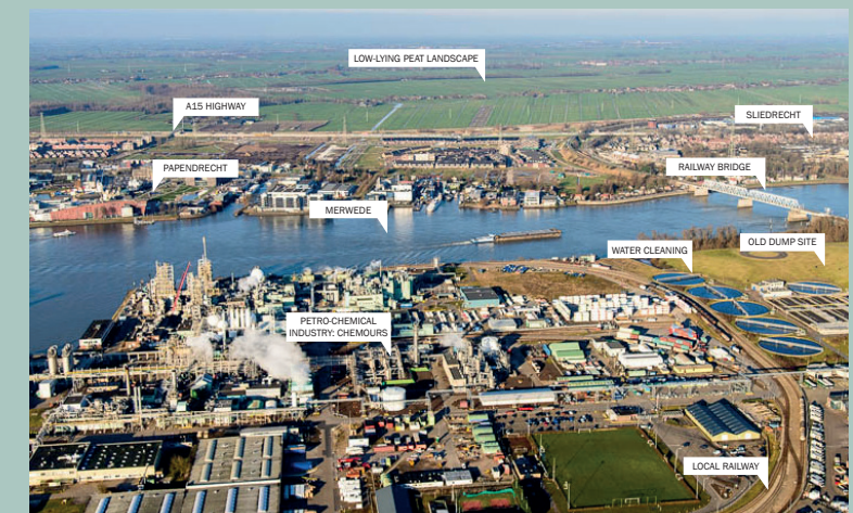
Figure 75: Petrochemical industry next to former waste dump site, which is replaced by a waste processing factory (Siebe Swart, 2018)
