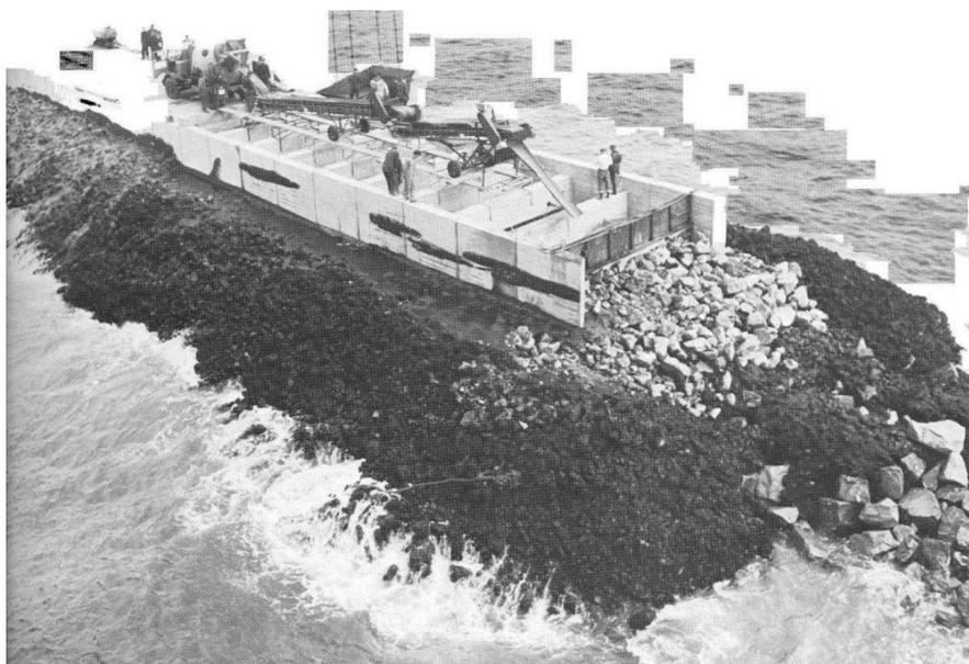
FIG. 6.2: *Asphalt cast to stabilize core during construction, Davidse (2012).*
