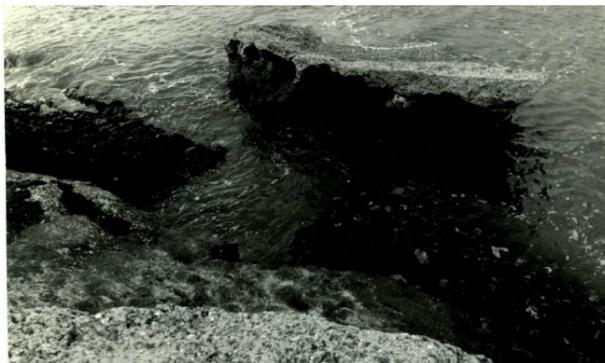
FIG. 1.4: *Damaged asphalt slab after summer storm of 1970, Davidse (2012).*
