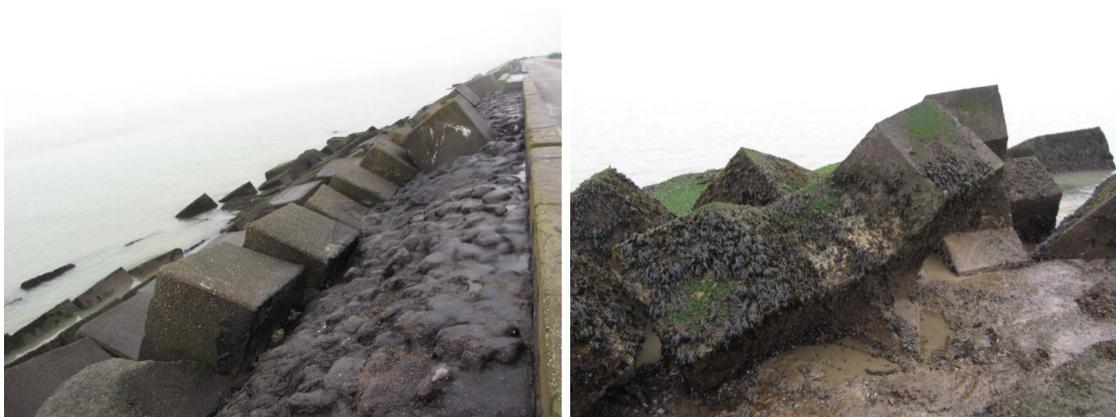
FIG. 6.3: *Armour units settling into the asphalt slab, pictures taken by author in January 2014.*
