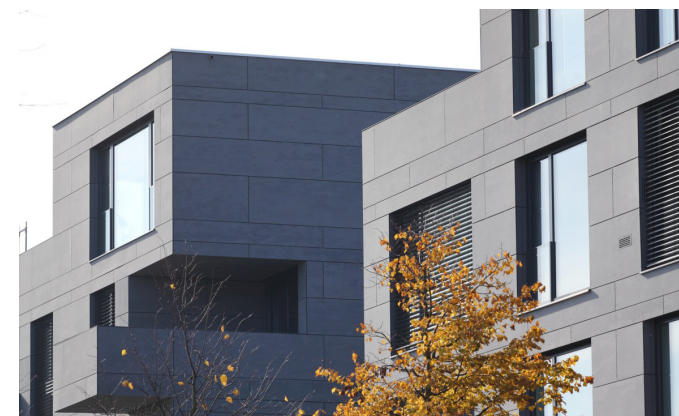
Think Green Building, Stuttgart by Bottega + Ehrhardt Architekten GmbH Using Equitone Fibre Cement Facades
