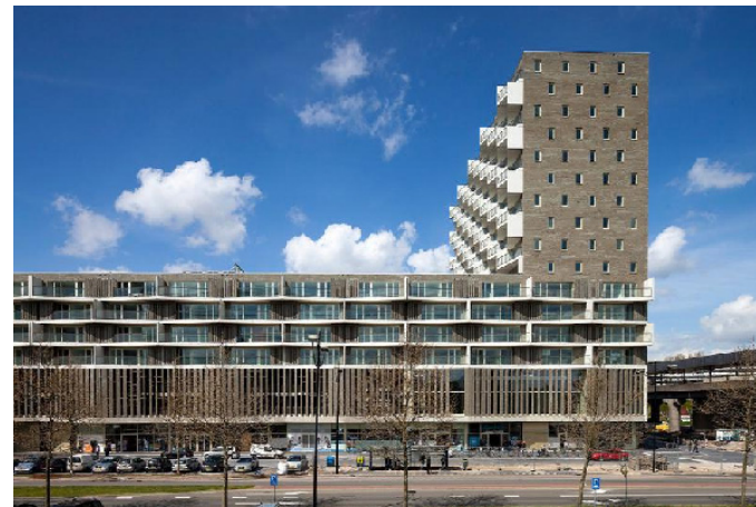
Figure 101. De Kameleon, 2012. Blijmermee, Netherlands. NL Architects
