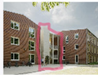
just a concrete block for the lift, nothing special
