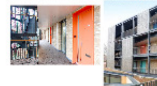
big wide flat columns that also serve as separators between each house, between spaces
