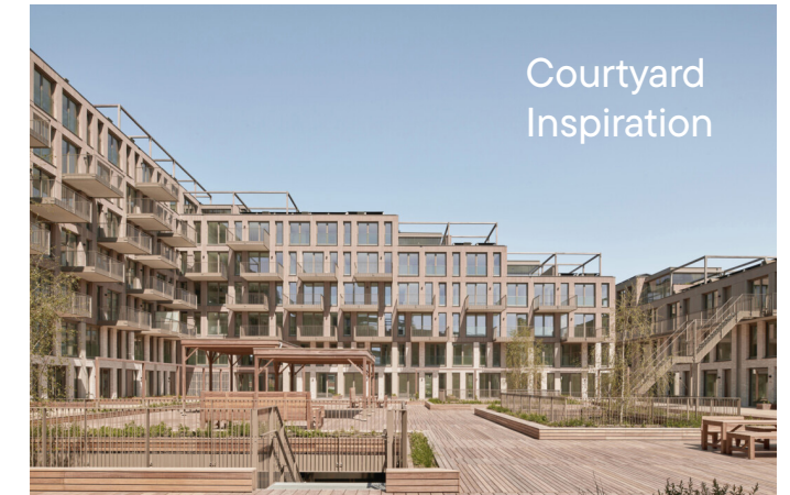
Figure 73. Leyhof Housing Complex, by Studio Ard Hoksbergen. The Hague, 2022.
