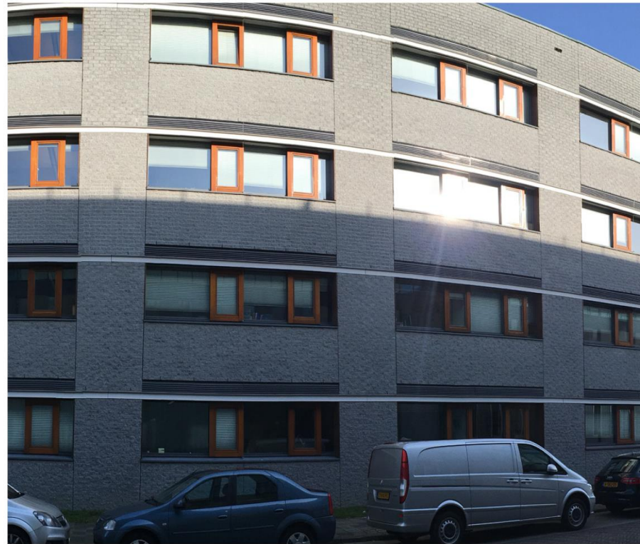
TPM Building facade
