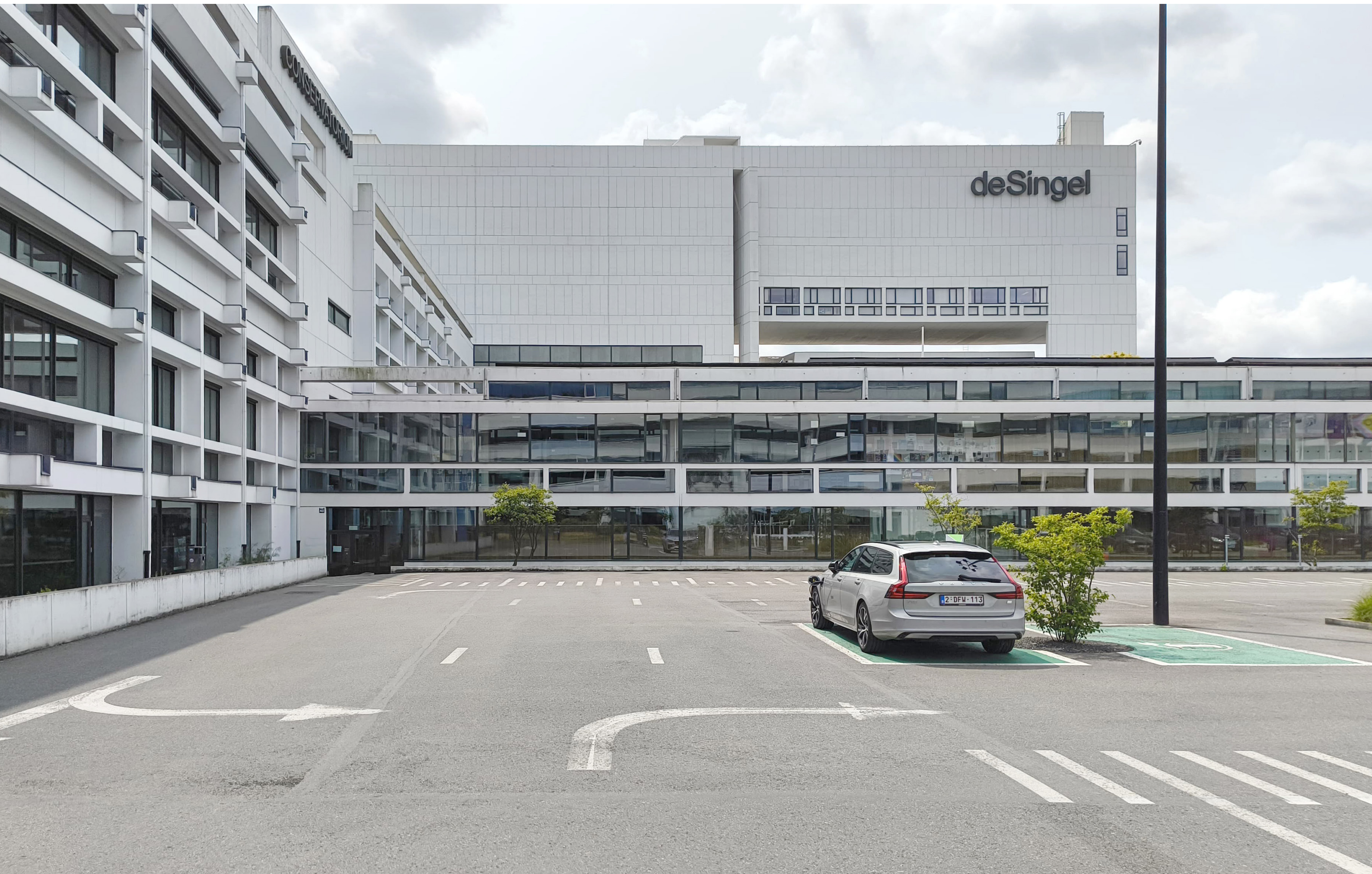
the corner facades
