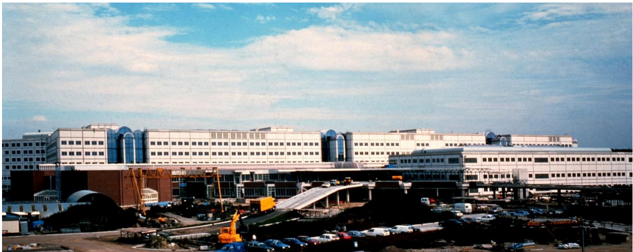
Figure 2: UMC hospital in Utrecht, EGM Architecten (1989). Photo from the Schokbeton archives @Heritage & Architecture.
