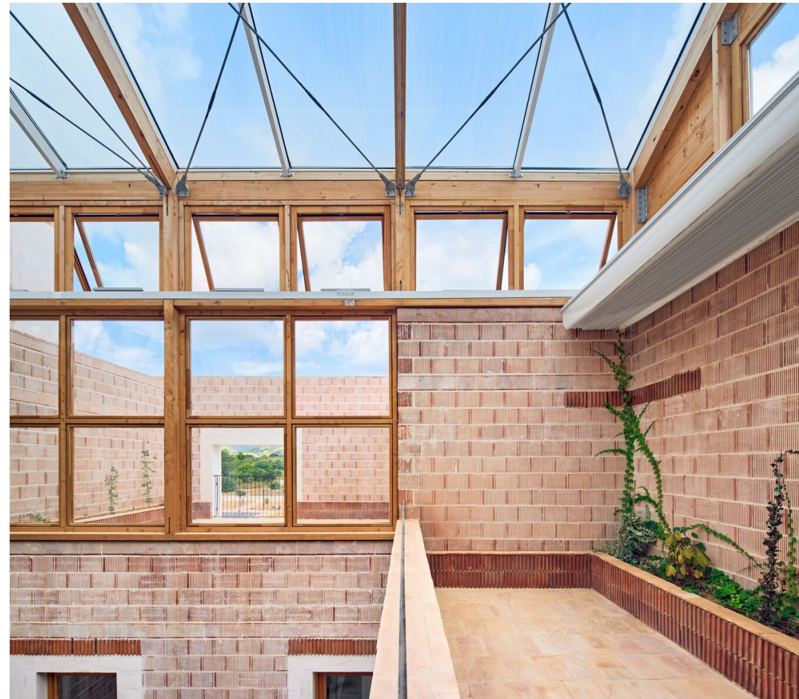
Figure 61: Thermal clay block filled with local soil.
