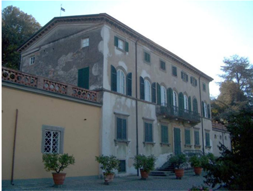
Fig. 2. Villa Burlamacchi, palace.
