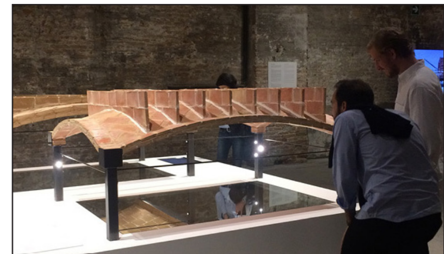
the spandrels solely transfer the floor load to the load bearing ceiling surface. similar to this reference of a vaulting system in tiles. (Block Research Group, 2016)
