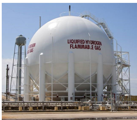
Figure 5.2: Liquid hydrogen storage. The sphere shape is chosen due to the minimal surface/volume ratio.
