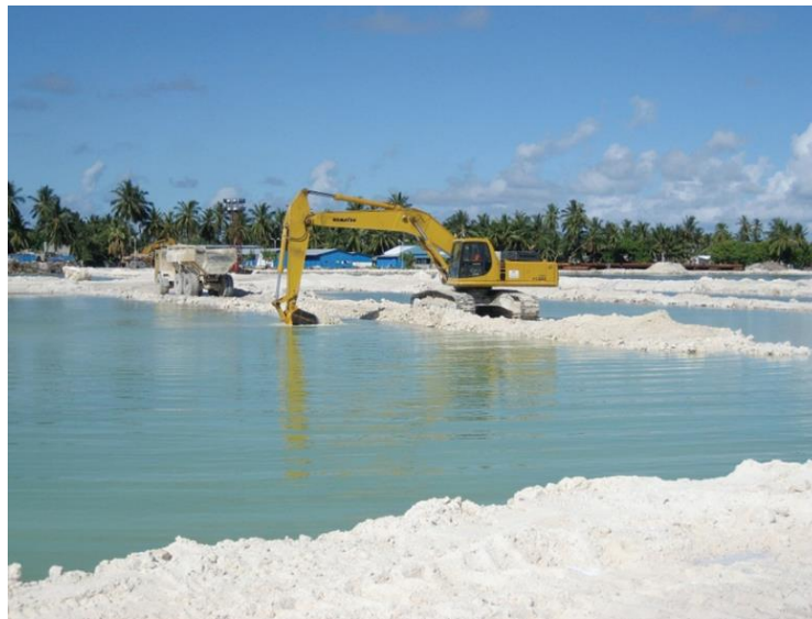
Figure 21 Truck dumping and profiling with excavators
