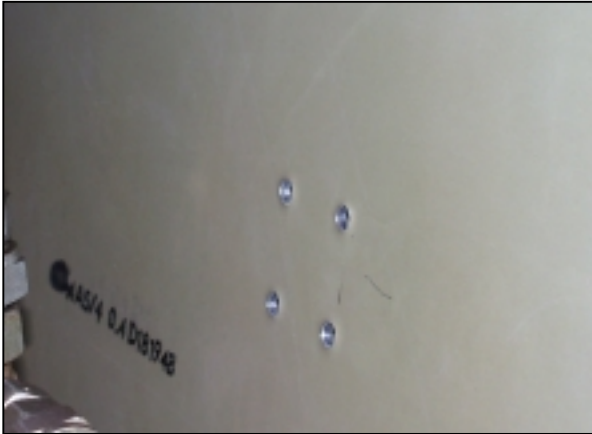
Figure 9.5. Bore holes at back side of panel
