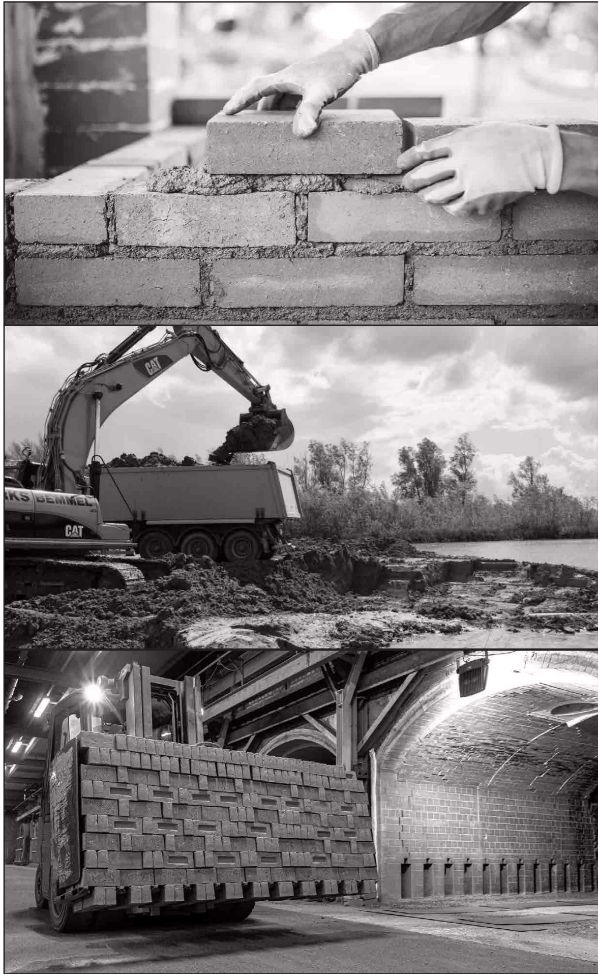
Main Construction Method Case Studies Research: Clay bricks with cement mortar
