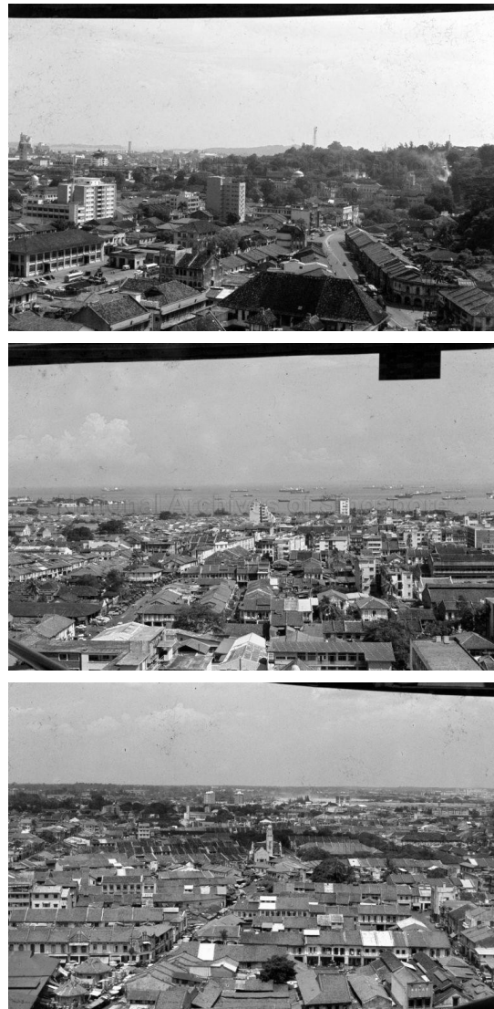
Fig. 45-47 View from viewing gallery, Selegie House, 1969. Source: National Archives of Singapore.
