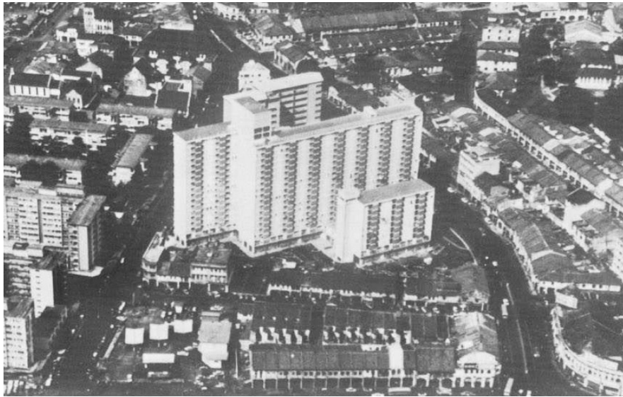
Fig. 41 Aerial photograph of Selegie House, c.1963. Source: HDB Annual Report 1963.
