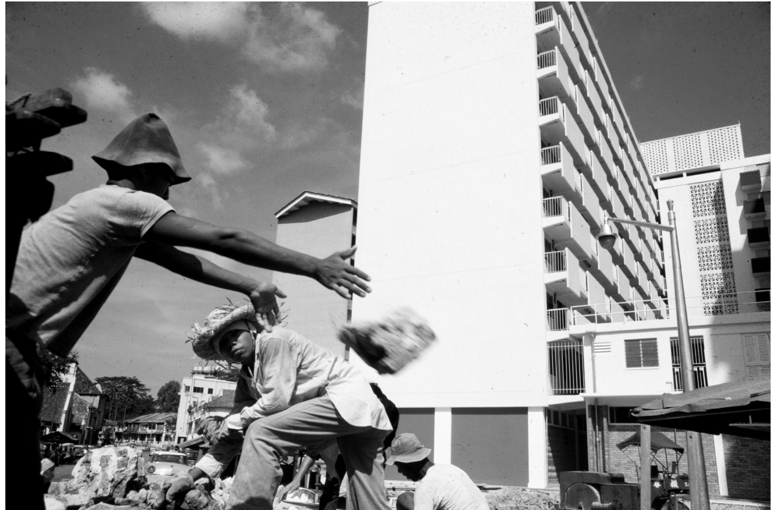
Fig. 42 Photograph of Selegie House and construction workers, c.1960s. Source: Brian Brake / National Museum of New Zealand.
