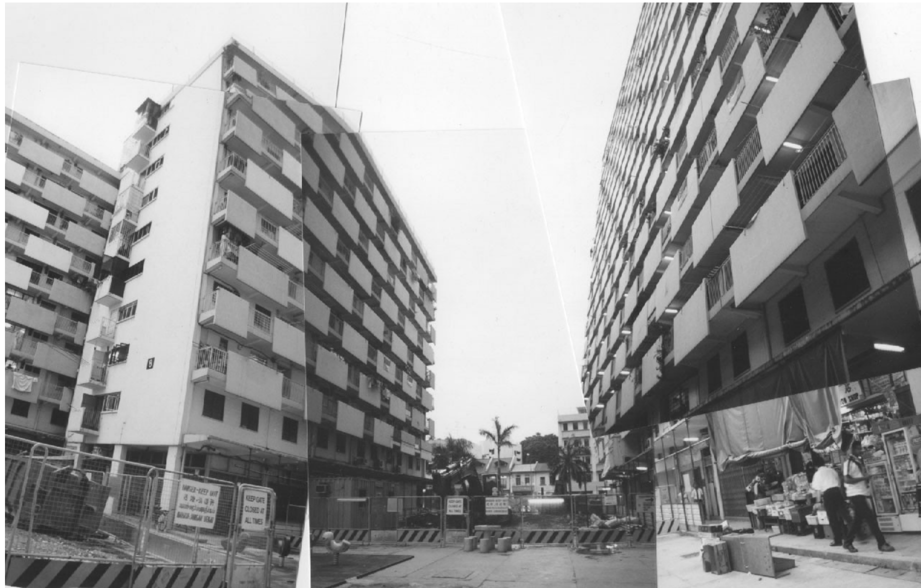
Fig. 51 Photograph showing demolition of commercial podium during upgrading works, c.2001. Source: Tan Kar Lin
