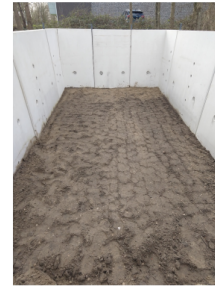
(b) Base layer with a 2% slope
