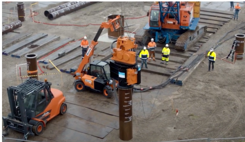
Figure 1: Pile installation at the GDP test site.
