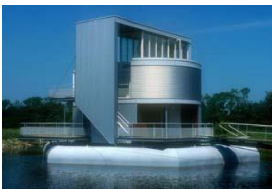
Figure 17: House on floating steel tubes 11
