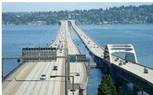
Figure 7: Homer M. Hadley Memorial Bridge (left) and Lacey V. Murrow Memorial Bridge (right) 7
