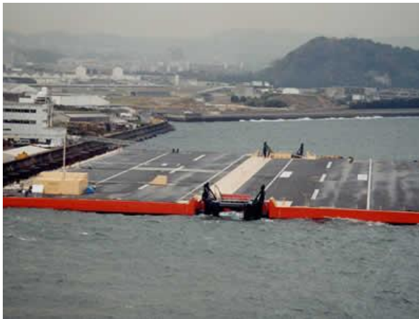
Figure 9: Installation of a mega-float IT base 9
