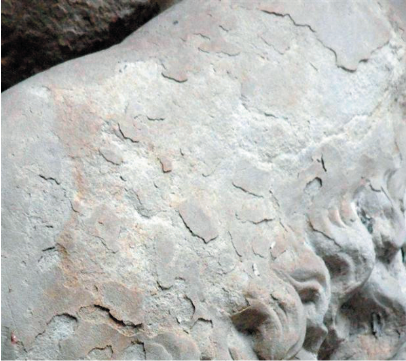
Figure 3: Detail of a natural stone showing scaling. In this situation a consolidation treatment is not suitable
