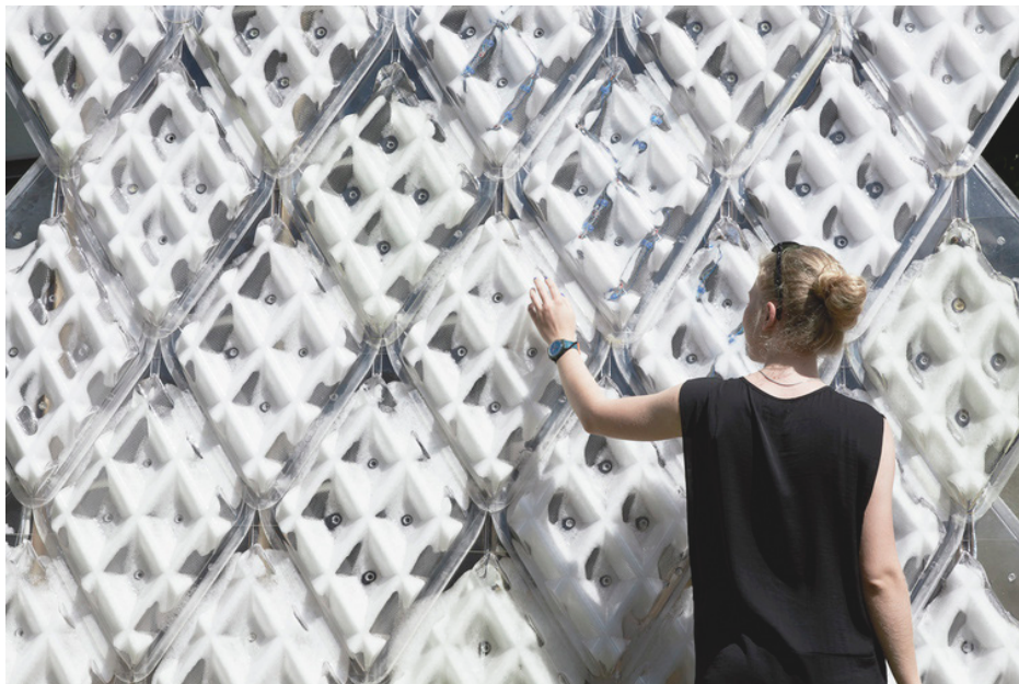
Figure 2.25: phase transition of paraffin in PCM façade project Source: from Phase Change Material (PCM) Façade , by Royal Danish Academy, 2018 ( https://bit.ly/3Vn4WiY )
