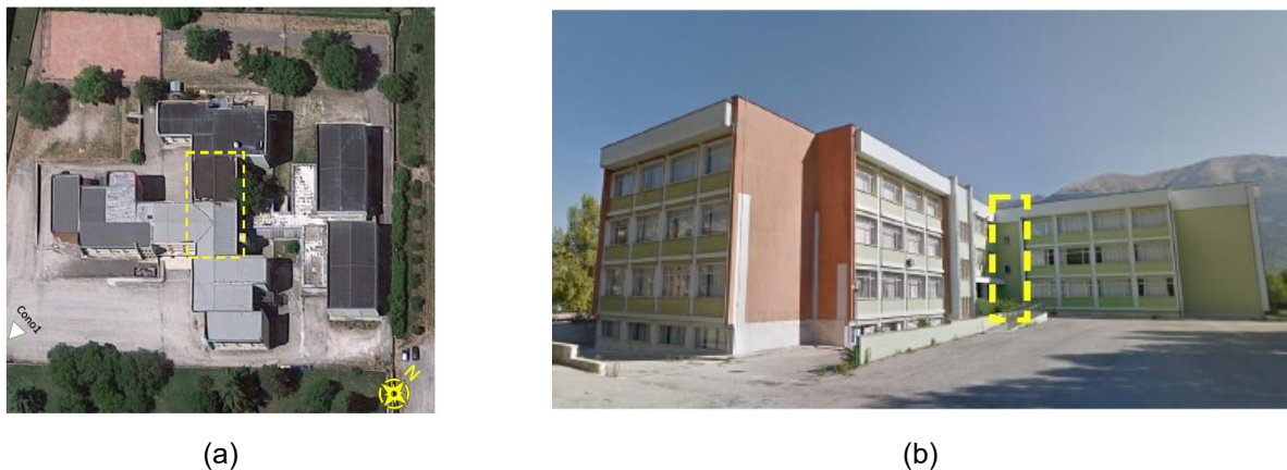
Figure 4. Case-study school building: (a) satellite view (Google Earth) and (b) a photo of the building (note: the analysed structural unit is highlighted in yellow).
