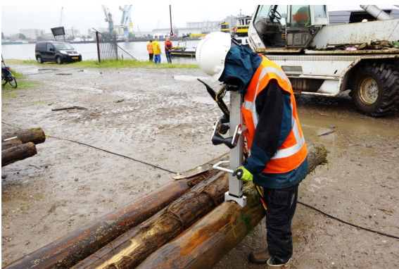
Figure 6: Microdrill in use on an excavated pile.
